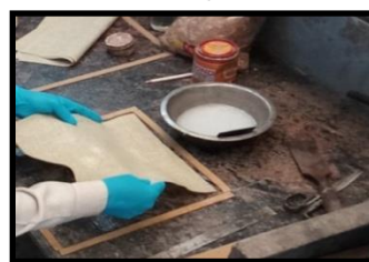
Fig2.4: Laying of Hemp
